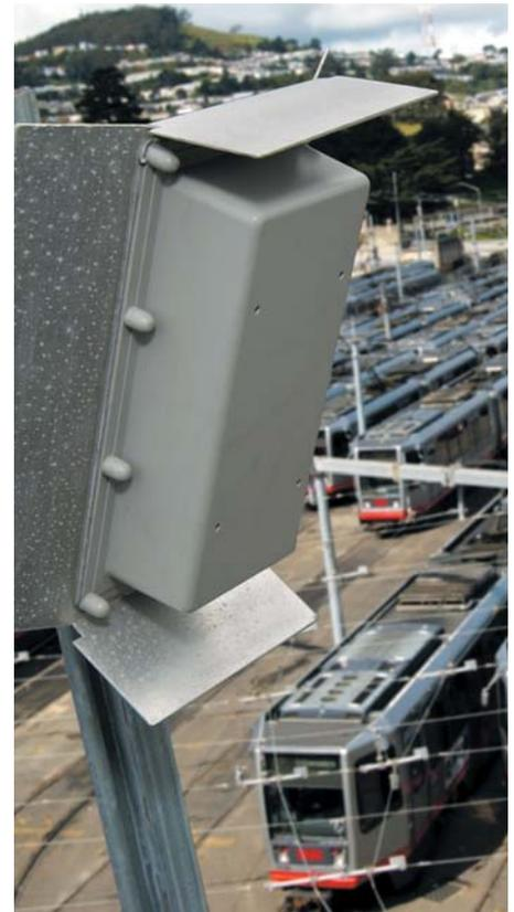
Wireless antennas mounted in Muni's light rail vehicle yard transmit video data from onboard March Networks 5308 MDVRs to a central server.
