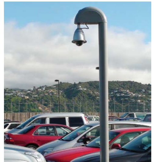
A water jet system remotely operated through March Networks' Site Manager software sprays and cleans the camera lenses located in the airport's outdoor car park.
